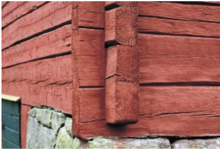
➤ Sustainable timber structure according to Swedish tradition, lifted above the ground moisture and protected by Falun red paint
