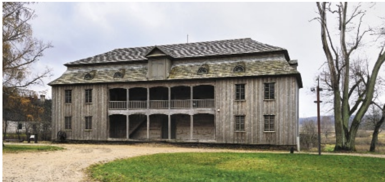
62 🏡 Kurtuvėnai Manor barn, built in the second half of the 18 th century (is now being reconstructed after a fire in 2001)
